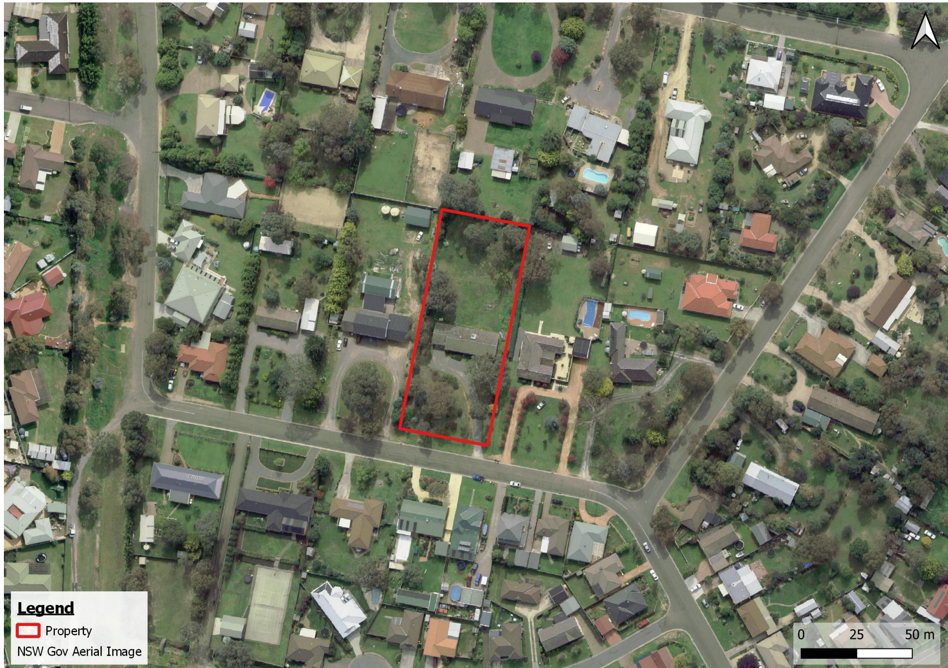
Figure 1-3: Aerial image of the property.
